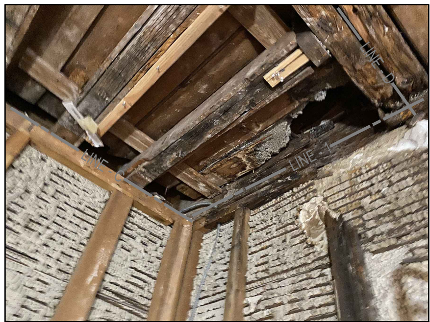
EXISTING CONDITION 3RD. FLOOR VIEWED FROM BELOW
