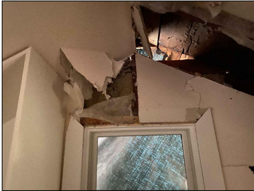
REPLACE DAMAGED FRAMING
