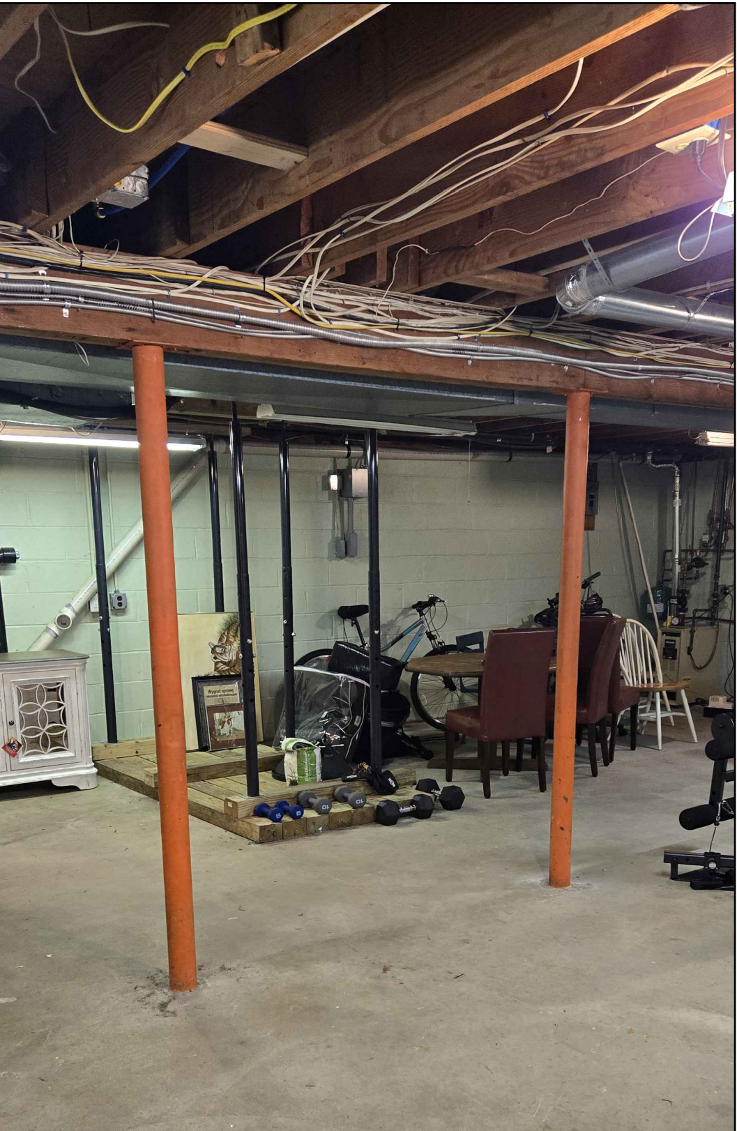
EXISTING CONDITION CLIENT-PROVIDED IMAGE
