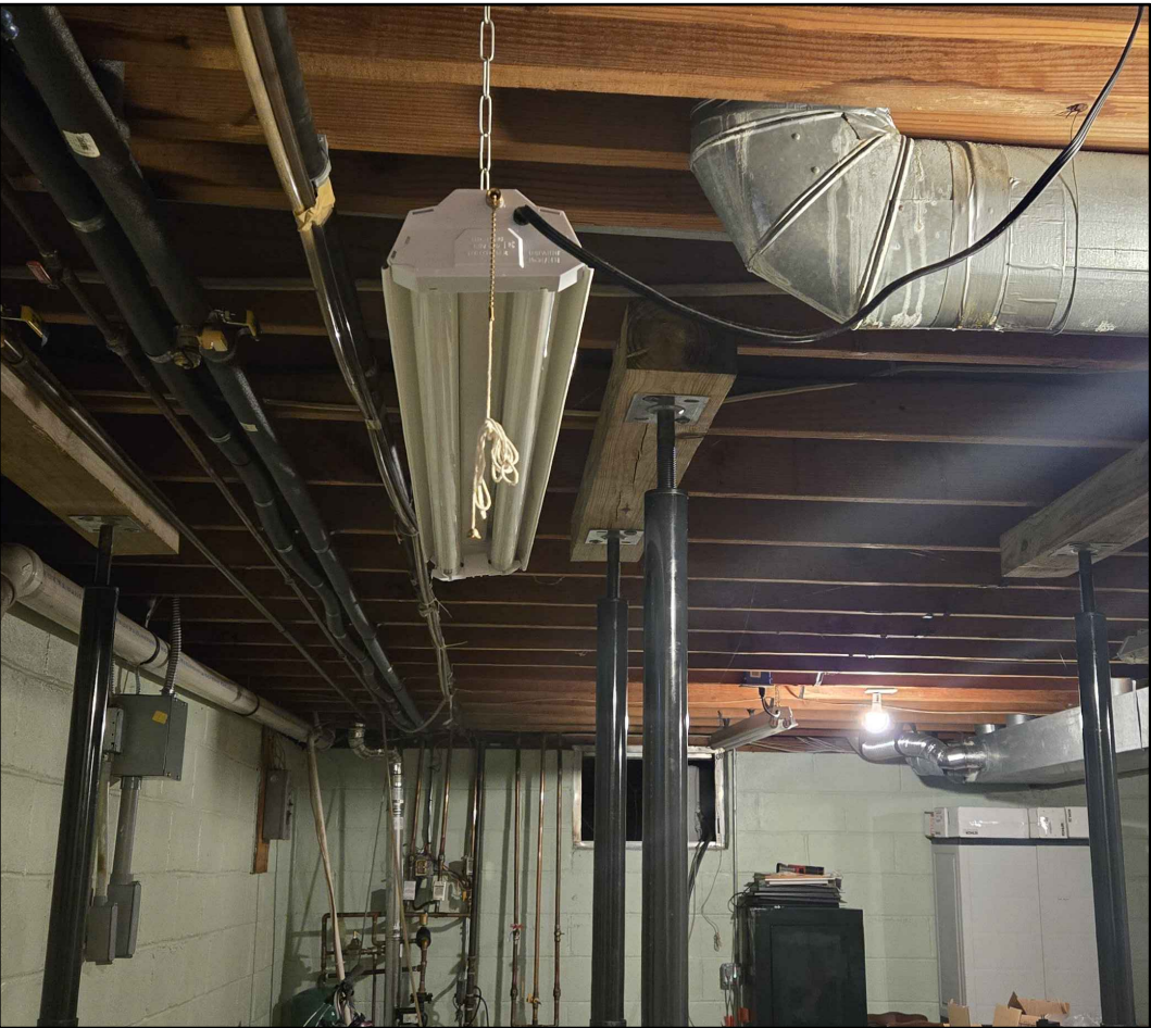
EXISTING CONDITION CLIENT-PROVIDED IMAGE
