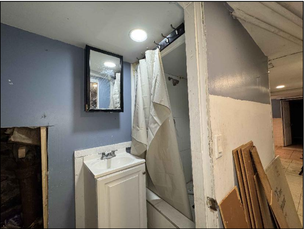
BATHROOM DEMOLISH FINISHES, FIXTURES AND WALLS; CAP ALL PIPES; RESTORE TO NON-HABITABLE STORAGE AREA
