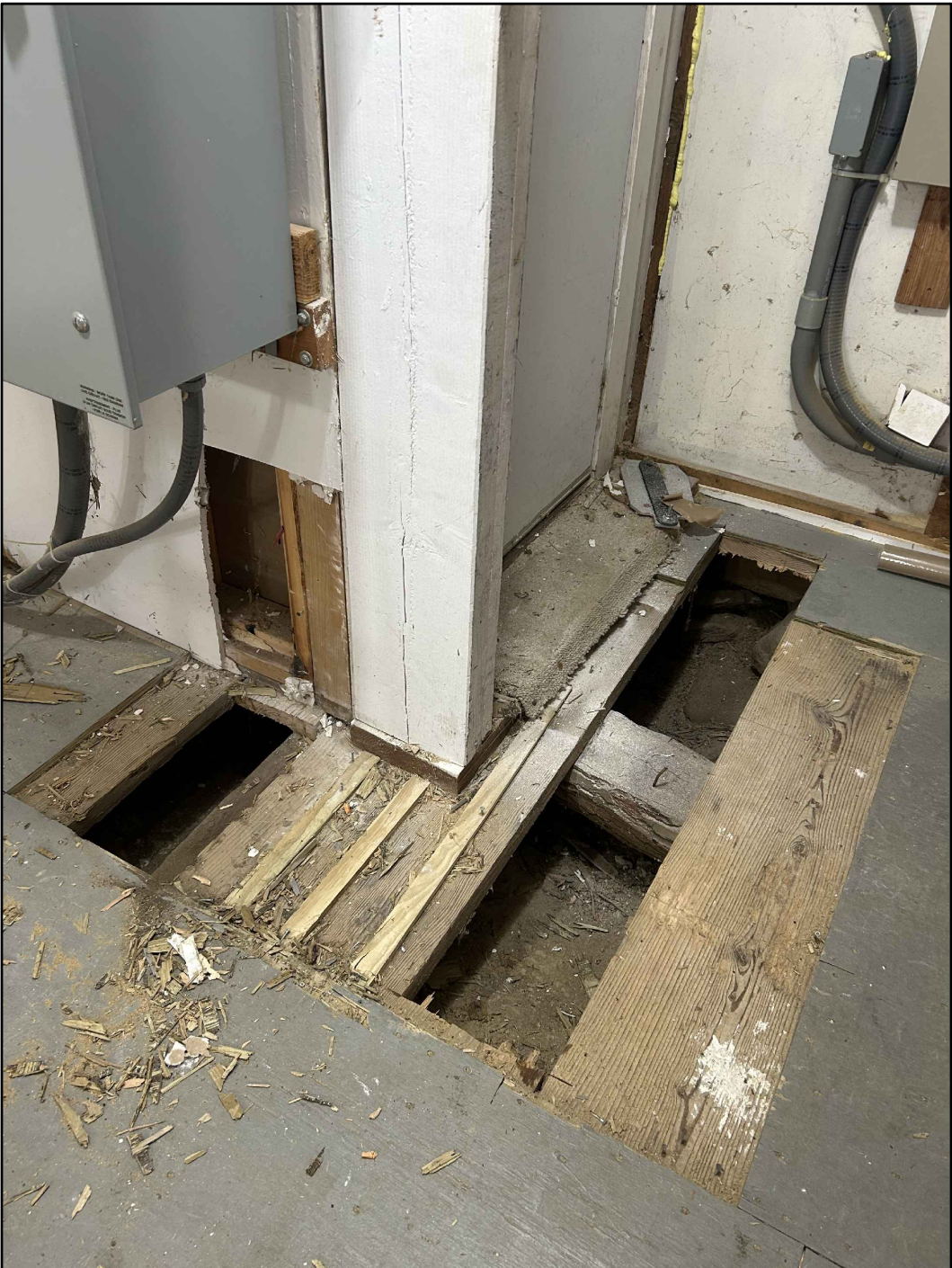
EXISTING CONDITION CLIENT-PROVIDED IMAGE
