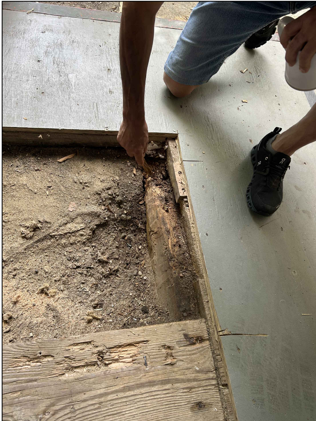
EXISTING CONDITION CLIENT-PROVIDED IMAGE
