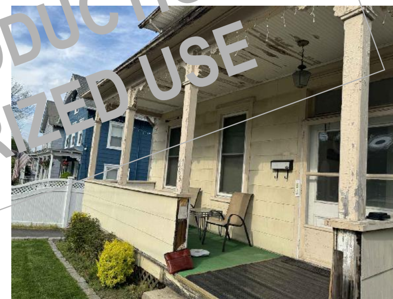
EXISTING PORCH REMOVE AND REPLACE FLOORING, GUARD RAIL & POSTS
