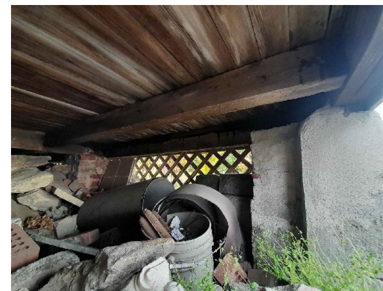
EXISTING PIER REMOVE AND REPLACE PIERS AND FOOTINGS
