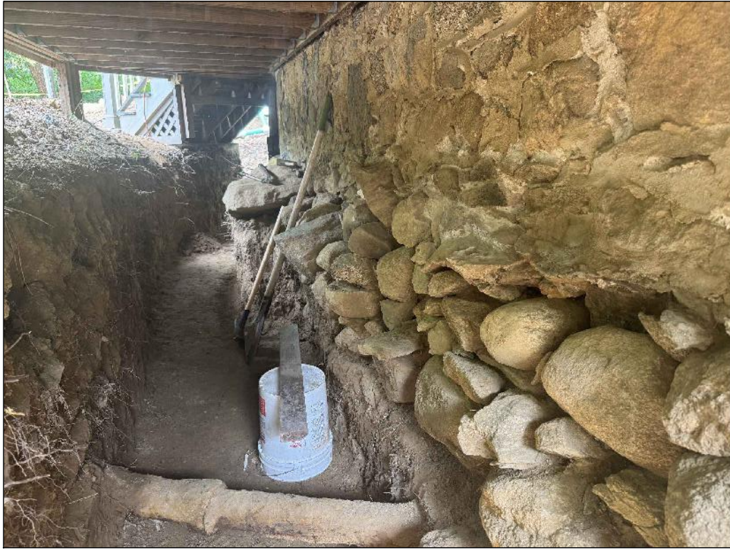
EXISTING CONDITION EXTERIOR OF RUBBLE MASONRY FOUNDATION; DRAIN BELOW WALL. 08.14.2025
