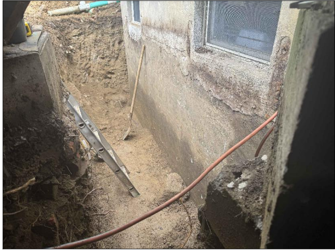
EXISTING CONDITION EXTERIOR OF CMU FOUNDATION 08.14.2025
