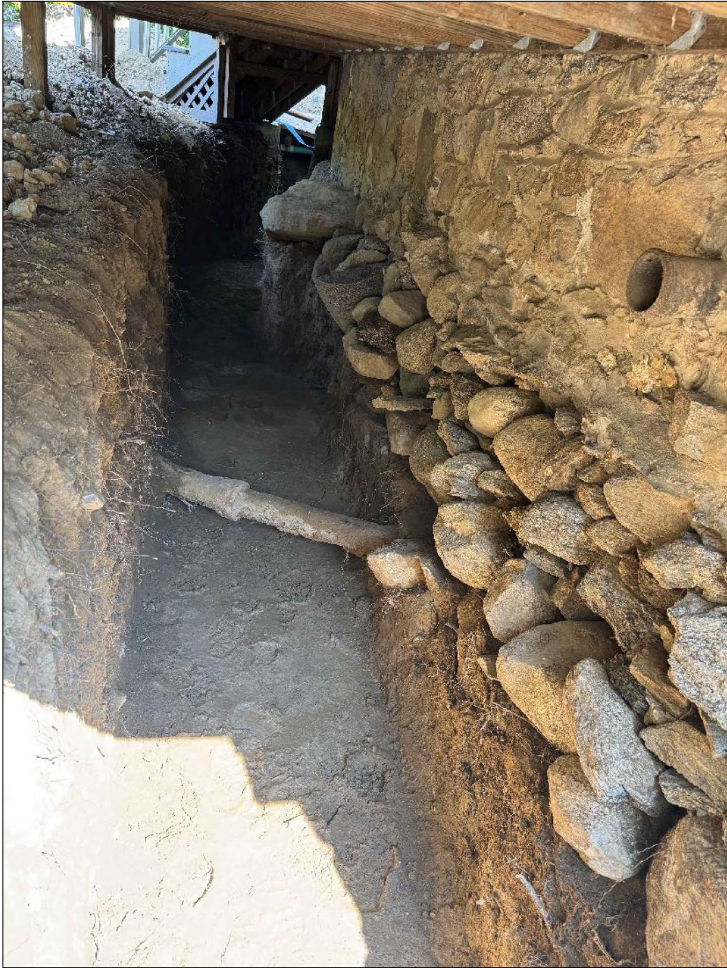
EXISTING CONDITION EXTERIOR OF RUBBLE MASONRY FOUNDATION 08.15.2025
