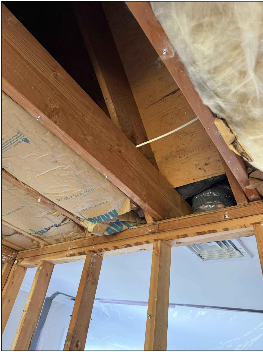
EXISTING CONDITION CLIENT-PROVIDED IMAGE
