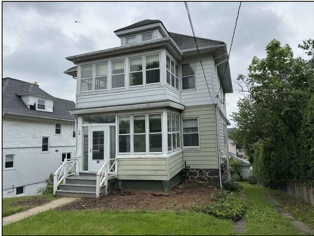
REBUILD FRONT "PORCH" EXISTING CONDITION 05.23.2025
