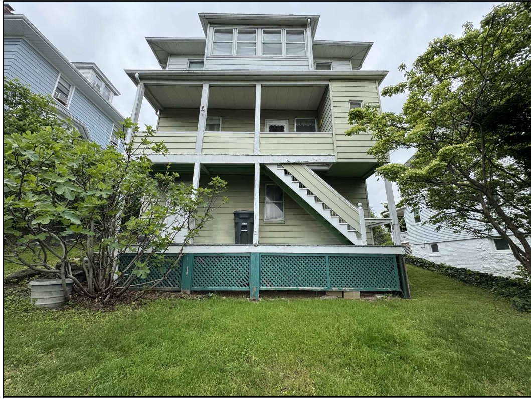
REBUILD REAR "PORCH" EXISTING CONDITION 05.23.2025
