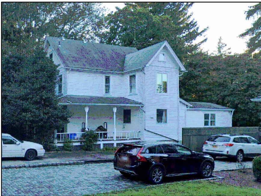
FRONT VIEW GOOGLE STREET VIEW
