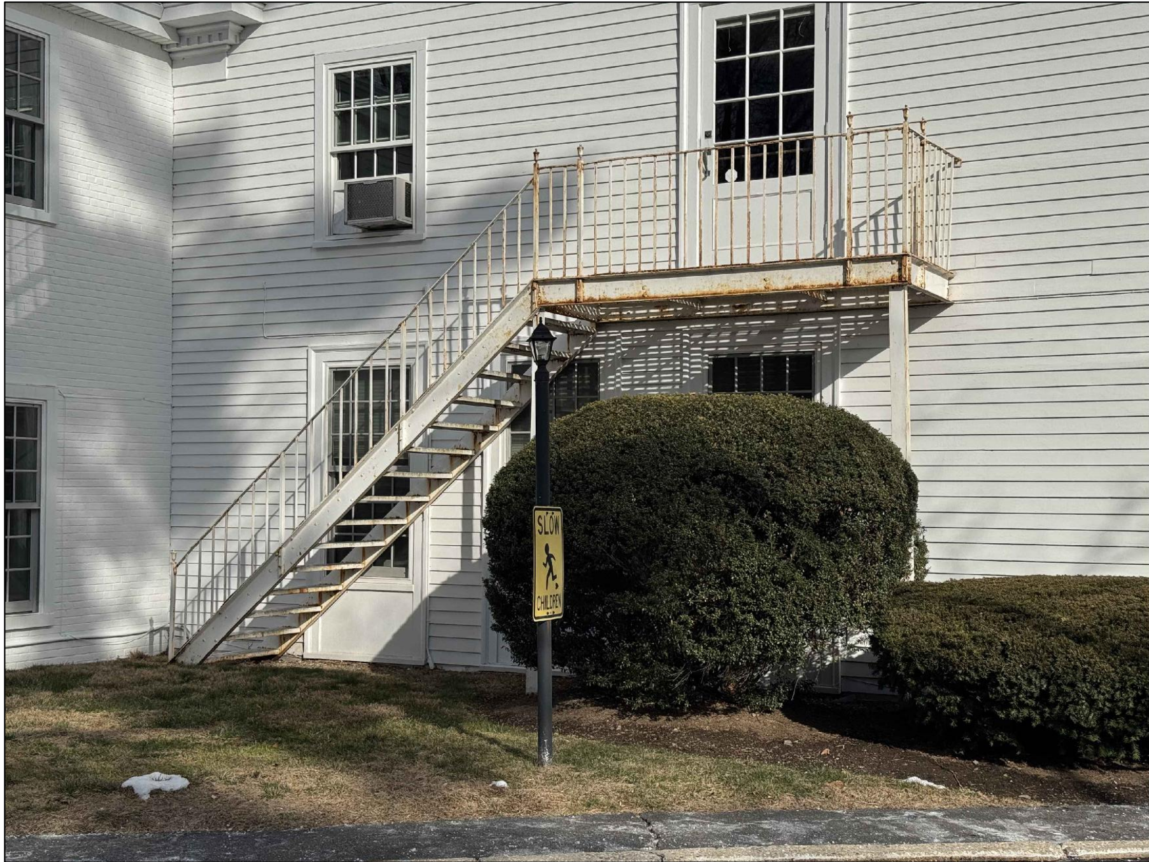
EXISTING FIRE ESCAPE - TO BE REPLACED 01.29.2025
