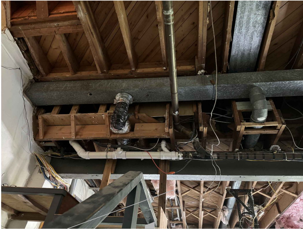
EXISTING CONDITION - SECOND FLOOR FRAMING 10.09.2024
