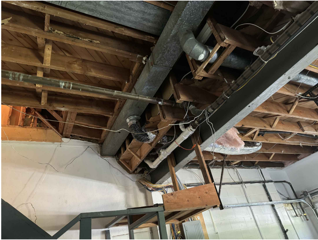
EXISTING CONDITION - SECOND FLOOR FRAMING 10.09.2024
